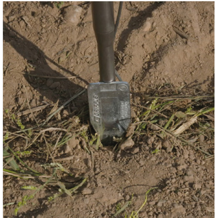
Anchor being driven into the ground
