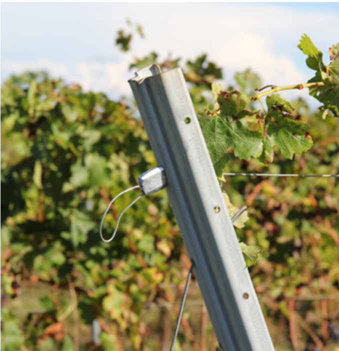
GP No.1 - Terminating trellis wire at a metal end post
