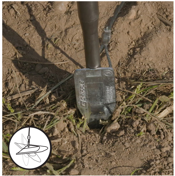
Anchor being driven into the ground
