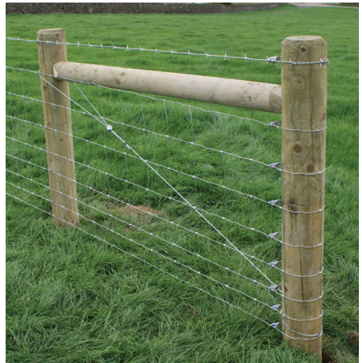
GPAK 3 - Bracing the end of a fencing run
