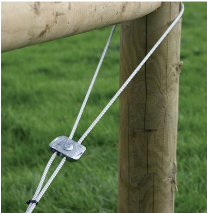
DPAK 6 - Installed as a H-Post brace
