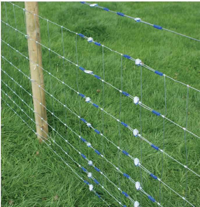
Gripple Plus Medium - Stock fence repair
